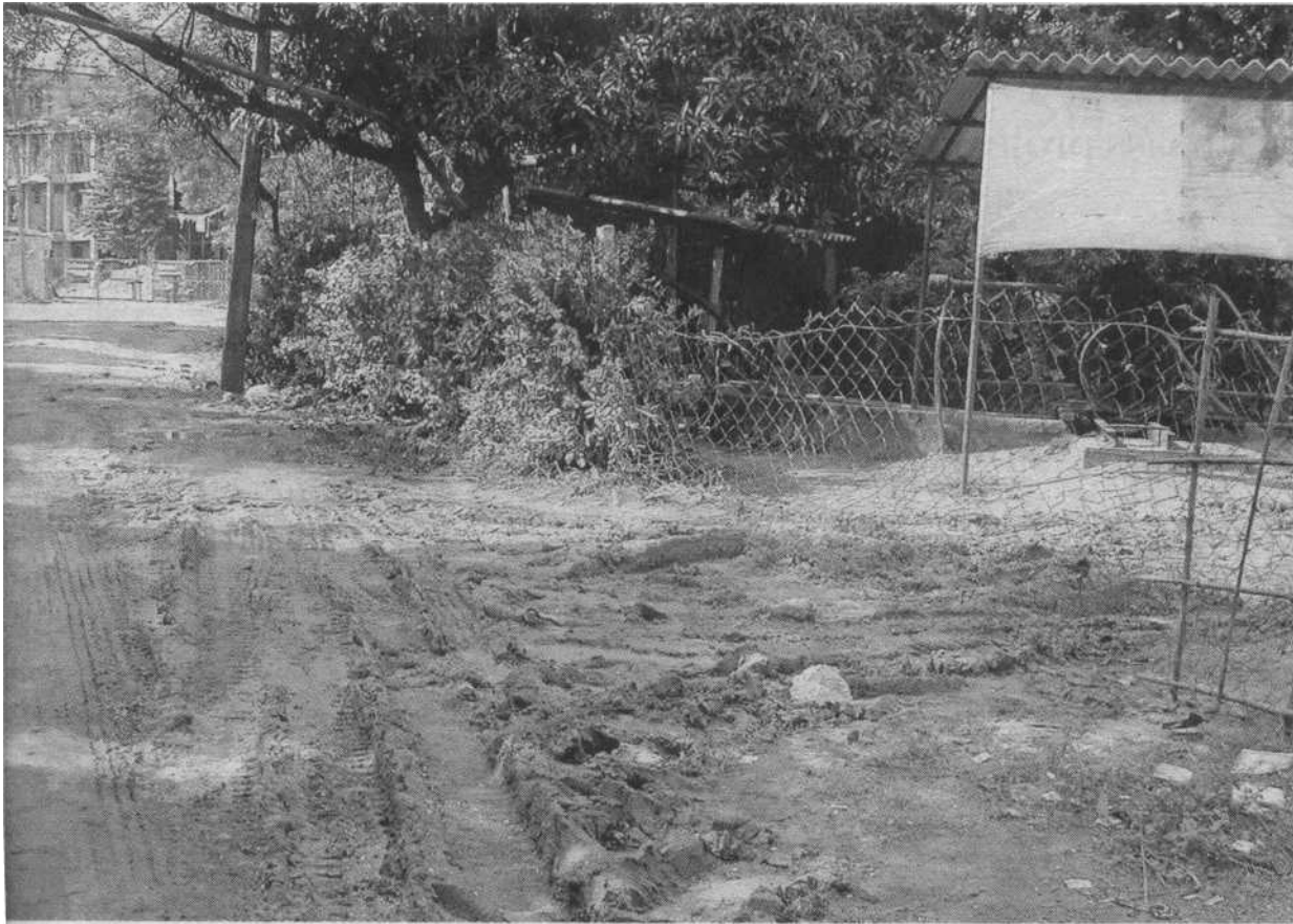
FALL-OUT: A road in Rose Nagar, which has a tell-tale sign of movement of lorries extracting water from farm wells.
