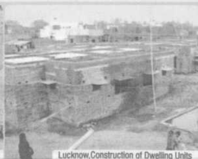
Lucknow, Construction of Dwelling Units
