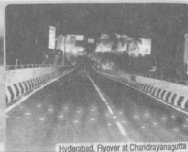
Hyderabad, Flyover at Chandrayanagutta
