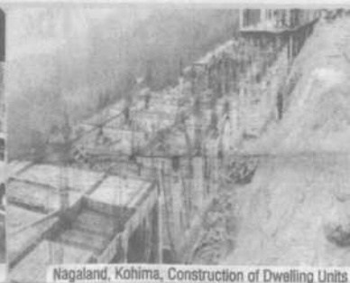
Nagaland, Kohima, Construction of Dwelling Units
