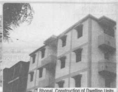
Bhopal, Construction of Dwelling Units
