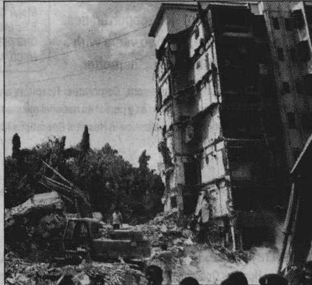
LIKE A PACK OF CARDS: The A wing of the Laxmi Chhaya building in Borivli collapsed last year, killing 29 people and injuring 18
